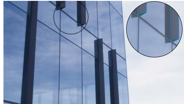
LIGHTLY TEXTURED GLASS VOLUMES UNIFY FACADE AND PROVIDE BACKDROP FOR PODIUM AND CORE EXPRESSIONS
