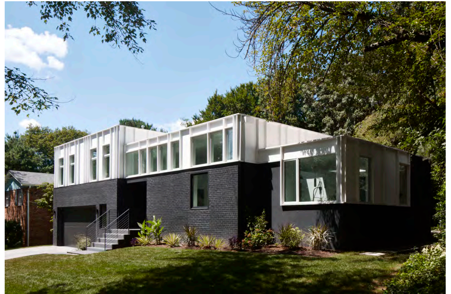
(above) Front view of Clerestory House
