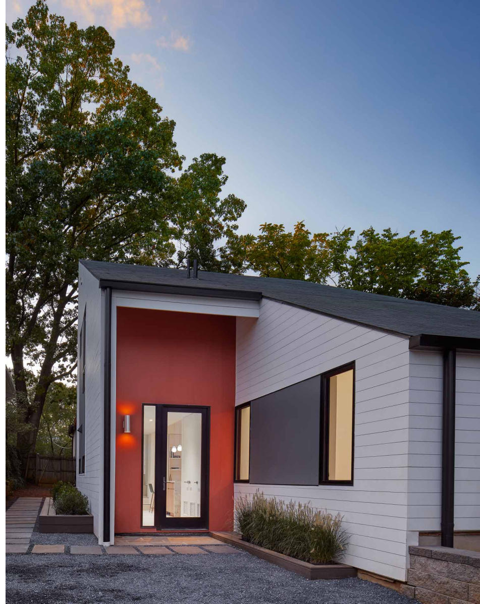
Entry from alley
