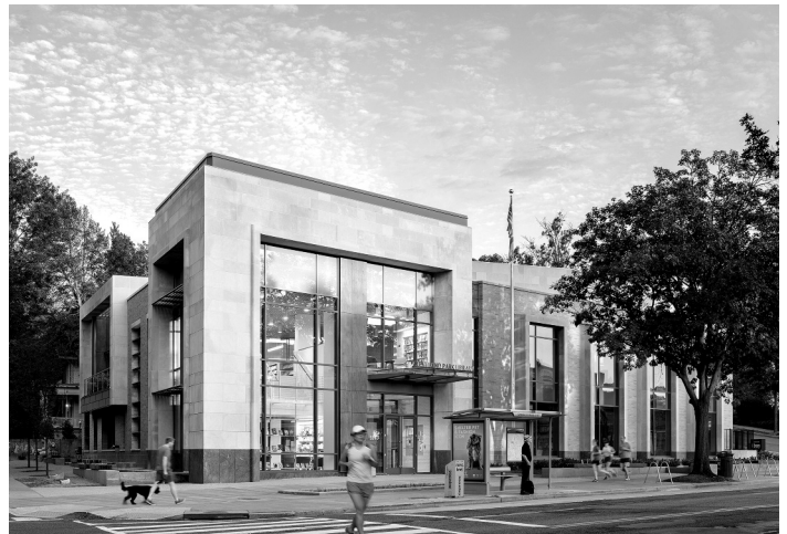
DC Public Library, Cleveland Park. Credit: Sarah Mechling, Perkins Eastman
